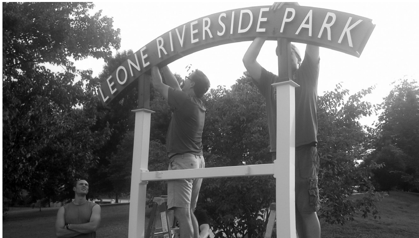
Seth supervises the Scotts as they remove the upper portion of the park sign. The sign is getting sanded, primed, painted, and some new info boards.
